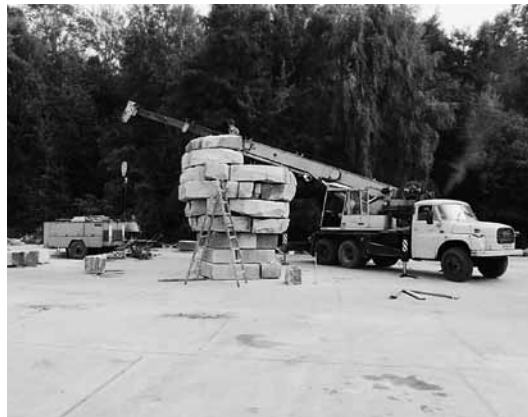
2 Instalace pískovcové Kvádrolavy sochaře Kurta Gebauera, 2002. / Installation of the sandstone Block-head by the sculptor Kurt Gebauer, 2002.
