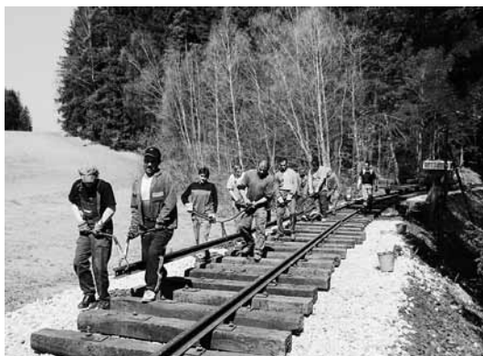
2 Oprava úzkokolejné trati, 2007. / Narrow-gauge railroad under repair, 2007. foto / photo Jan Šatava (1, 2)
